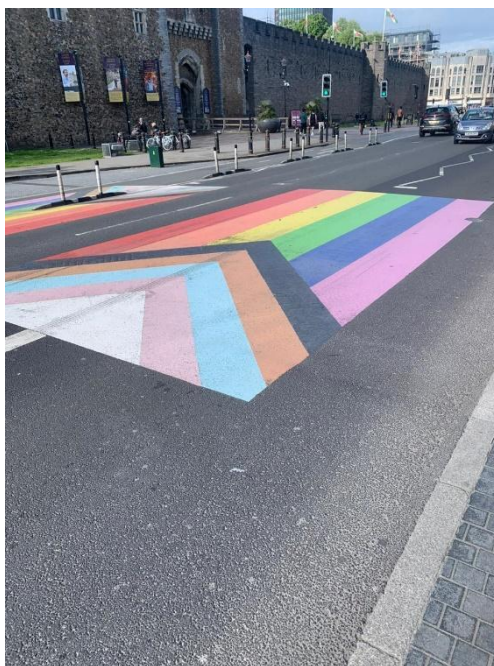
Figure 5.1 Trans pedestrian crossing. Source: author's file (Cardiff, Wales).
